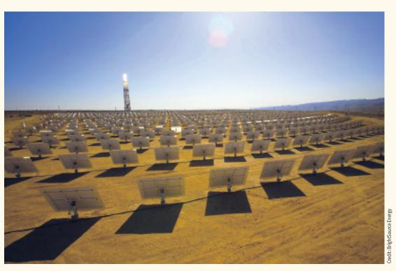
When completed, Ivanpah will look similar to this solar array in Israel. The smaller, flat mirrors are more efficient, simpler to manufacture, and cost less to install than parabolic mirrors used in solar troughs.
